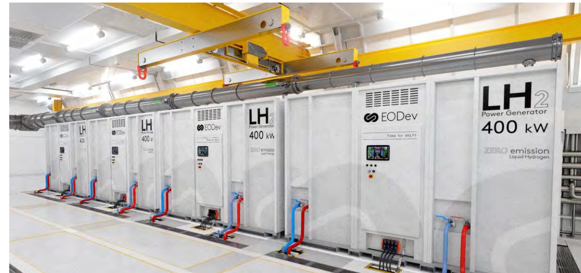
3D views of the EOConcept Fuel Cell Room integrating EODev modules based on a new generation of Toyota fuel cells delivered in 2026
